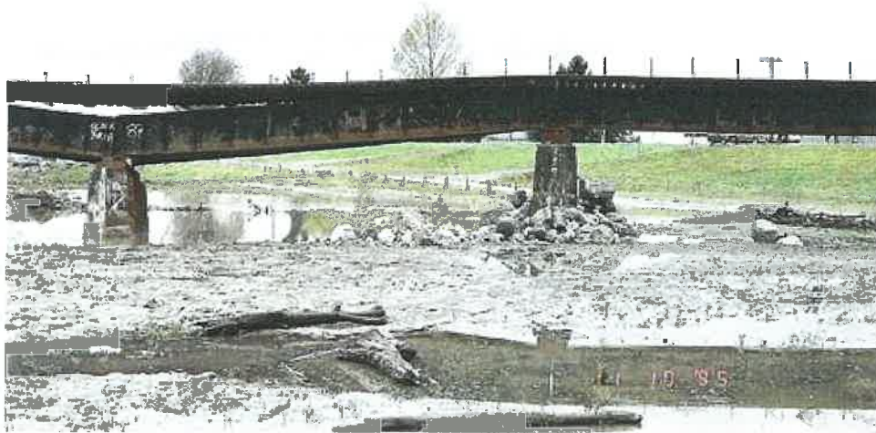
BNSF Skagit River Bridge, November, 1995
